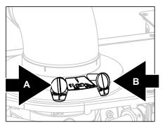
A – Flue gas sample point B – Air intake sample point Figure 15.2.a
